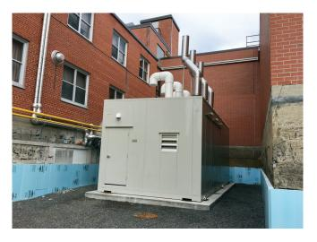
Preserving space inside the hospital, the self-contained hot water boiler plant was shipped on skids to the job site, pre-assembled and factory tested, and located outside adjacent to the existing boiler plant.
